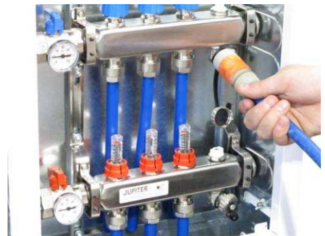
Connect pressure test equipment to upper return valve. Before connecting pressure test to the in-situ hose lock, pump some water out through the connecting pipe to avoid pumping unnecessary air into system. Before opening return valve with cap bring pressure up to approx. 5 bar.
