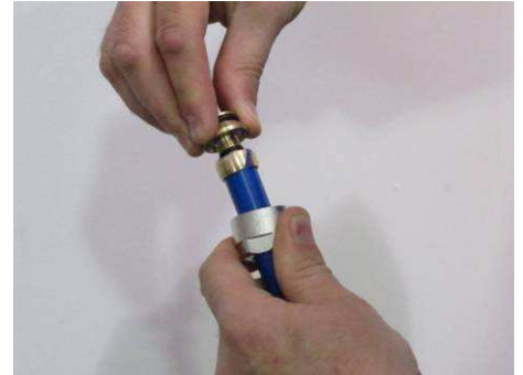
Place nut and brass split ring over pipe before inserting Eurokone fitting
