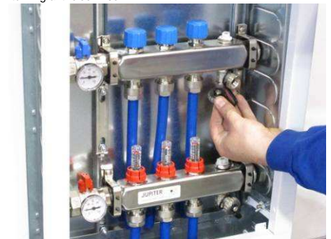
Open fill and drain valve using key on the back of cap
