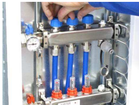
Re-open all blue caps on upper manifold prior to pressure testing.
