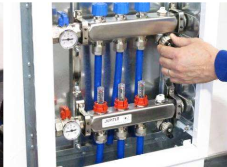
Once completed decrease pressure to 2 bar and then close return valve using cap. Release remaining pressure before removing test equipment from manifold. Remove testing equipment and close cap.
