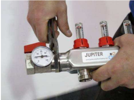
Fix isolating valves to the manifold – insert separately packed thermostatic dial into slot on flow & return valves
