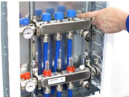
Close all blue caps on the return manifold except for circuit to be filled
